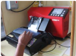
✓ Helium Leak Detection Test
